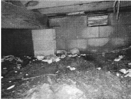
Crawlspace views. No moisture barrier in crawlspace.
