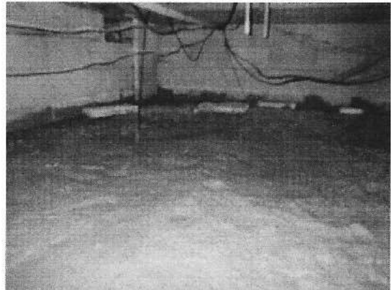
Crawlspace views. No moisture barrier in crawlspace.
